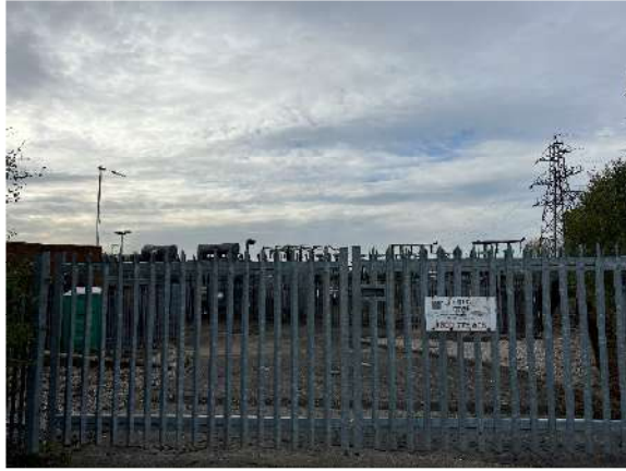
Plate 33 - Area 11 Substation adjacent east boundary
