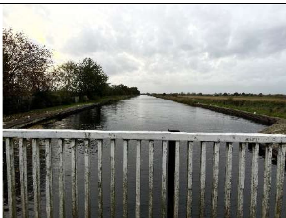
Plate 31 - Area 8 Mauds Bridge over Canal looking west
