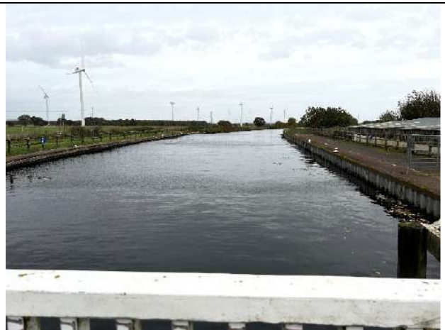
Plate 30 -Area 8 Mauds Bridge over Canal looking east
