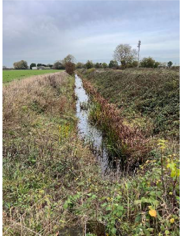
Plate 2 – Area 3 North Idle Drain looking North from Plains Drain junction bridge. Peat Deposits
